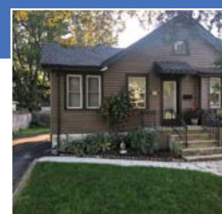
EXTERIOR Roofing, Siding & Windows
