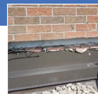
FOUNDATIONS Water Damage & Brick Repair
