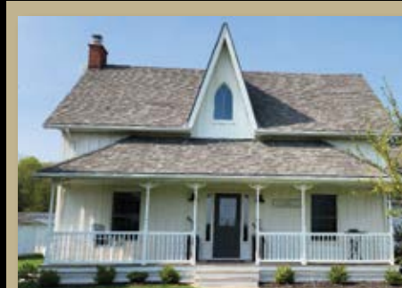
83399 Southgate Rd. 8, Southgate
