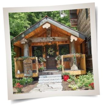
patina. Chinking – the use of mortar to seal joints between logs – was only included on this house as a 'throw-back' aesthetic. Log ends are dovetailed; no nails were used on the log house. David built and stained the wooden window boxes on the upper and lower levels himself. Filled with a profusion of colourful red geraniums and assorted greenery, they add a sensational splash of colour.
