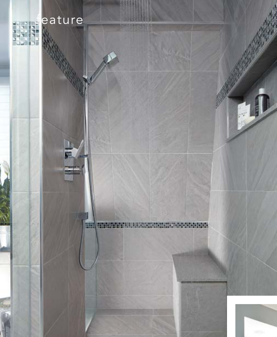
ABOVE: A rainhead shower and subtly-sloped floor keep water contained in the doorless shower, no matter how much splashing goes on. The bench and shelf feature the same quartz as the countertop. RIGHT: Andrew went into the master bath renovation without a plan, opting to demolish first and see what space they had to work with. They chose a Victoria + Albert free-standing bath because it's spacious and yet has a small footprint. FAR RIGHT: Building on a Dior Grey (Benjamin Moore) accent wall, the master bedroom is classic and timeless. Window coverings by Alexanian Carpet & Flooring. Window seats by Foamland.
