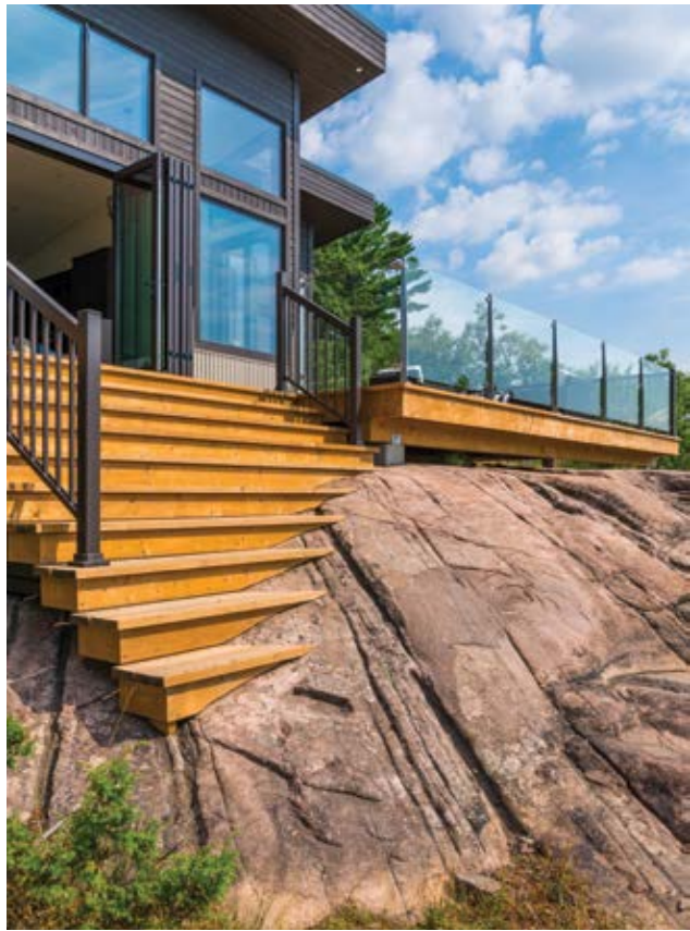
Wooden stairs ascending the granite slope to the cottage were individually sculpted to fit snugly against the rock.
